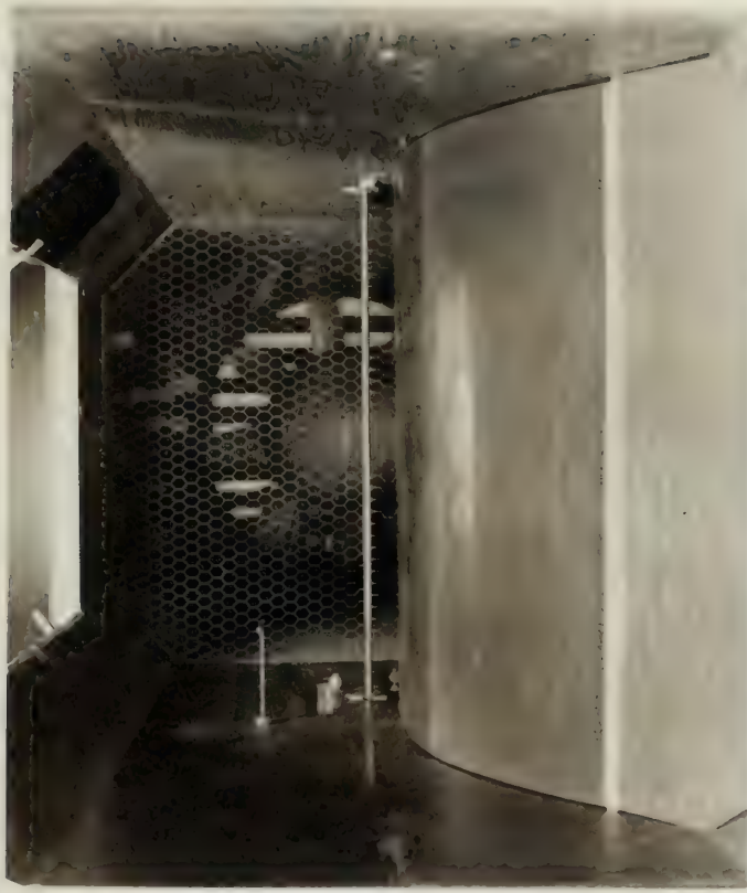
a. Test section showing airfoil and barrier
